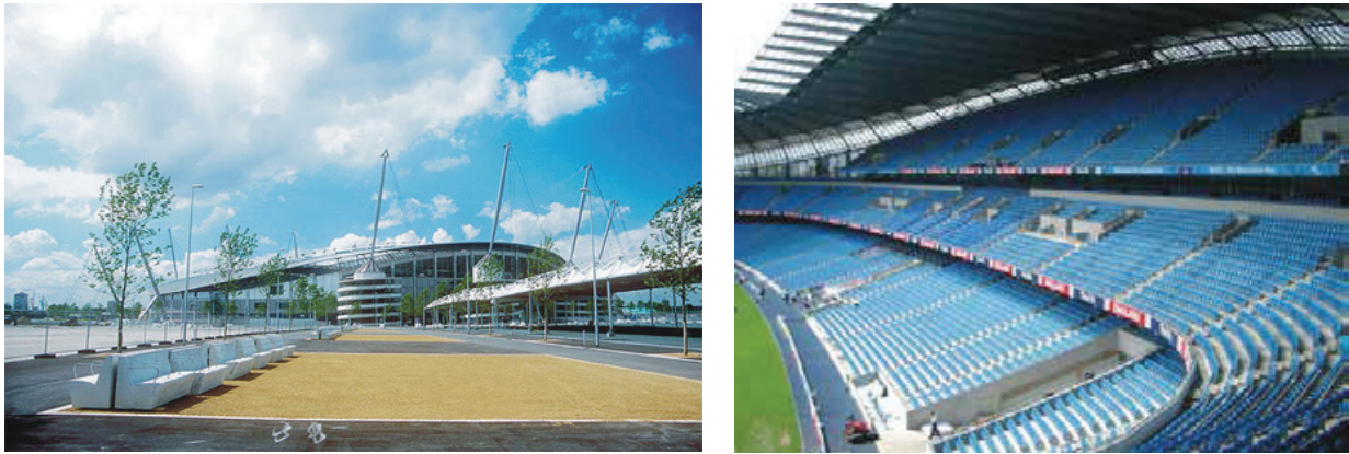
Figure 1: External and Internal Views of the Stadium.
